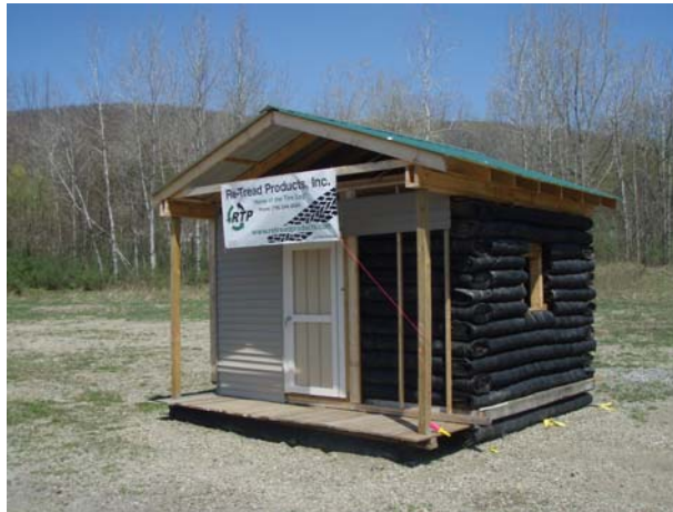
This small "log cabin" was built using Re-Tread's tire logs. Photo submitted
